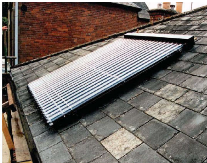
Solar hot water panel (evacuated tube system)
